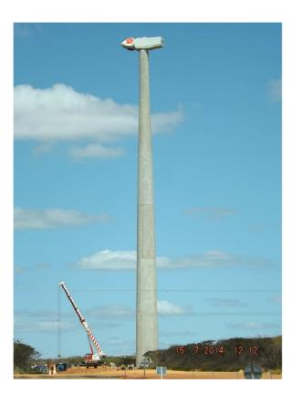
A new stage has just been accomplished on the first of its worksites, the site of Areia Branca, where the first nacelle has been put-up on top of the 120 metre tower.
