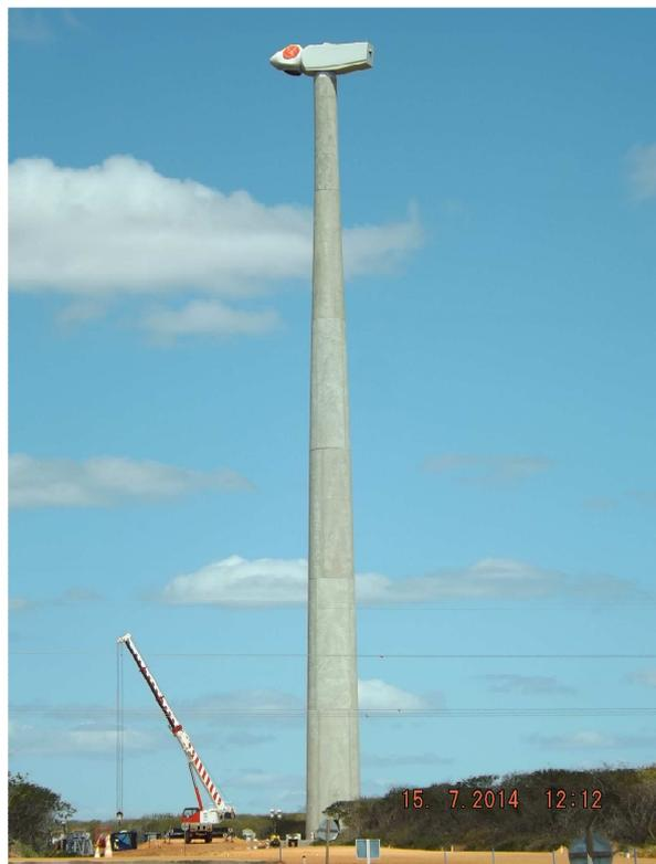
A new stage has just been accomplished on the first of its worksites, the site of Areia Branca, where the first nacelle has been put-up on top of the 120 metre tower.
