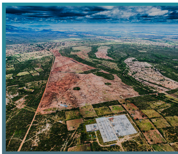
Bolobedu power plant in South Africa, whose annual output should enable to avoid over 237,000 tonnes of CO 2 emissions.
